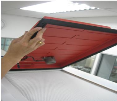
Figure 5.7. Lifting & Removing the Damper
